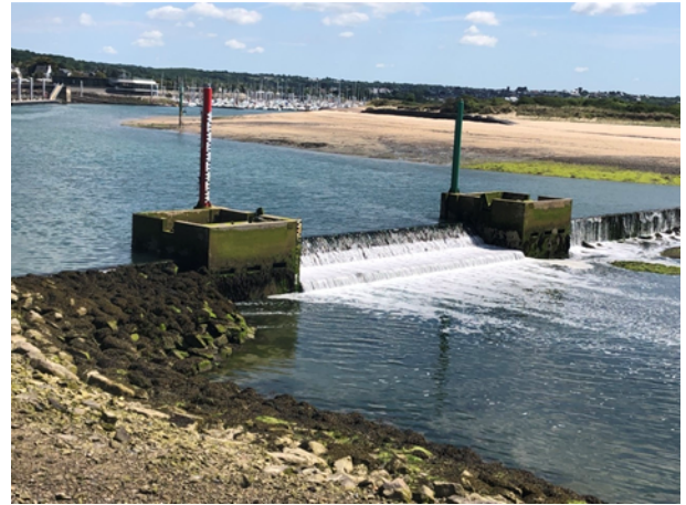
Carteret: the new sill
