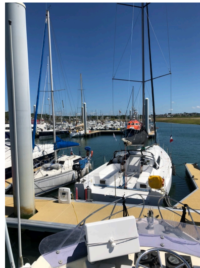
The new pontoons at Carteret
