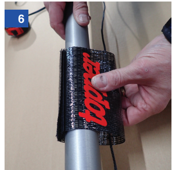
And then wrap the mylar strap around the boom
